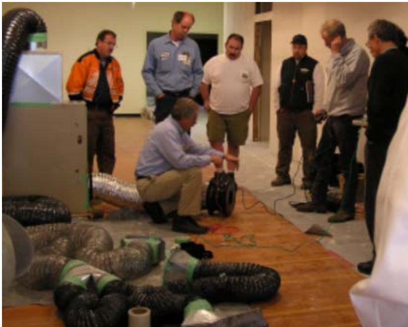
Doug Beaman shows a group of contractors how to perform a duct leakage test.
